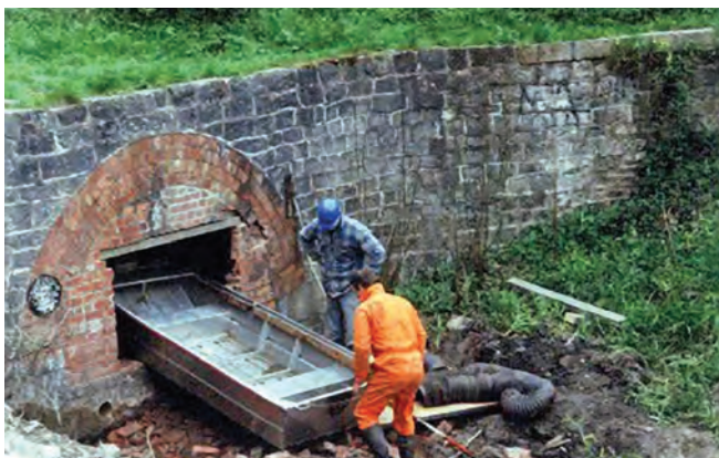
Tunnel inspection in the winter of 2002/3. Photo Mike Sampson
